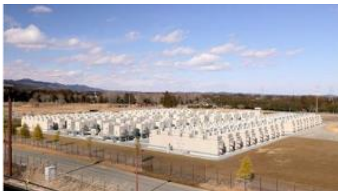
Figure 84: Picture of the 40 MW and 40 MWh energy storage system in Fukushima, Japan (Ref. 48).
