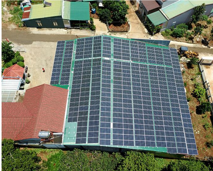
PV solar rooftop in Dak Nong province (135 kWp)
