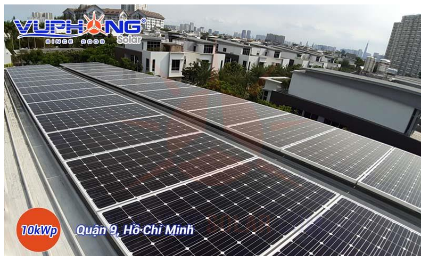
PV solar rooftop in District 9, Ho Chi Minh city (10.08 kW p )
